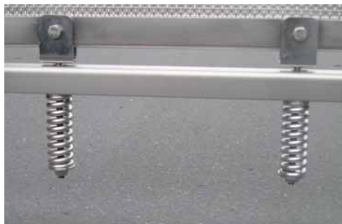
Intermediate fixing: Wire connector
